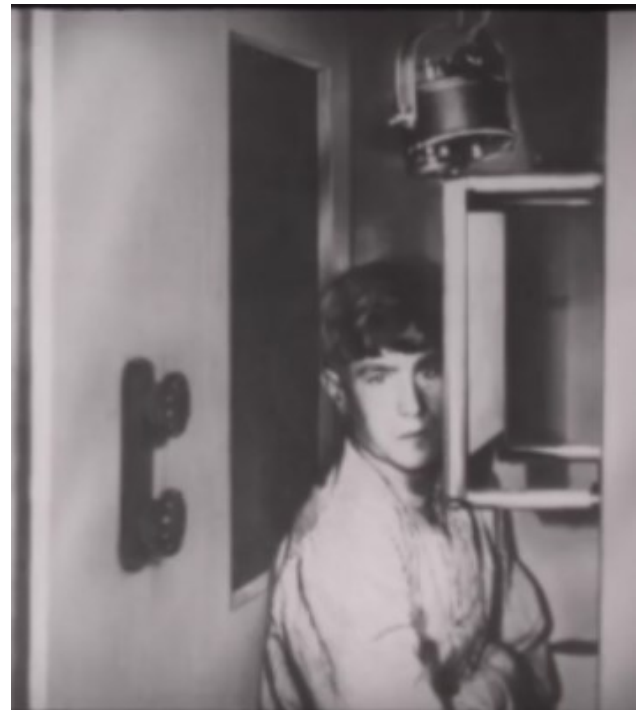
Figure 2: The recording setup used for the 1935 film. The light rectangular panel is the fluoroscope screen and the camera (not shown) is located to the right. Notice the large microphone mounted at the top right.
